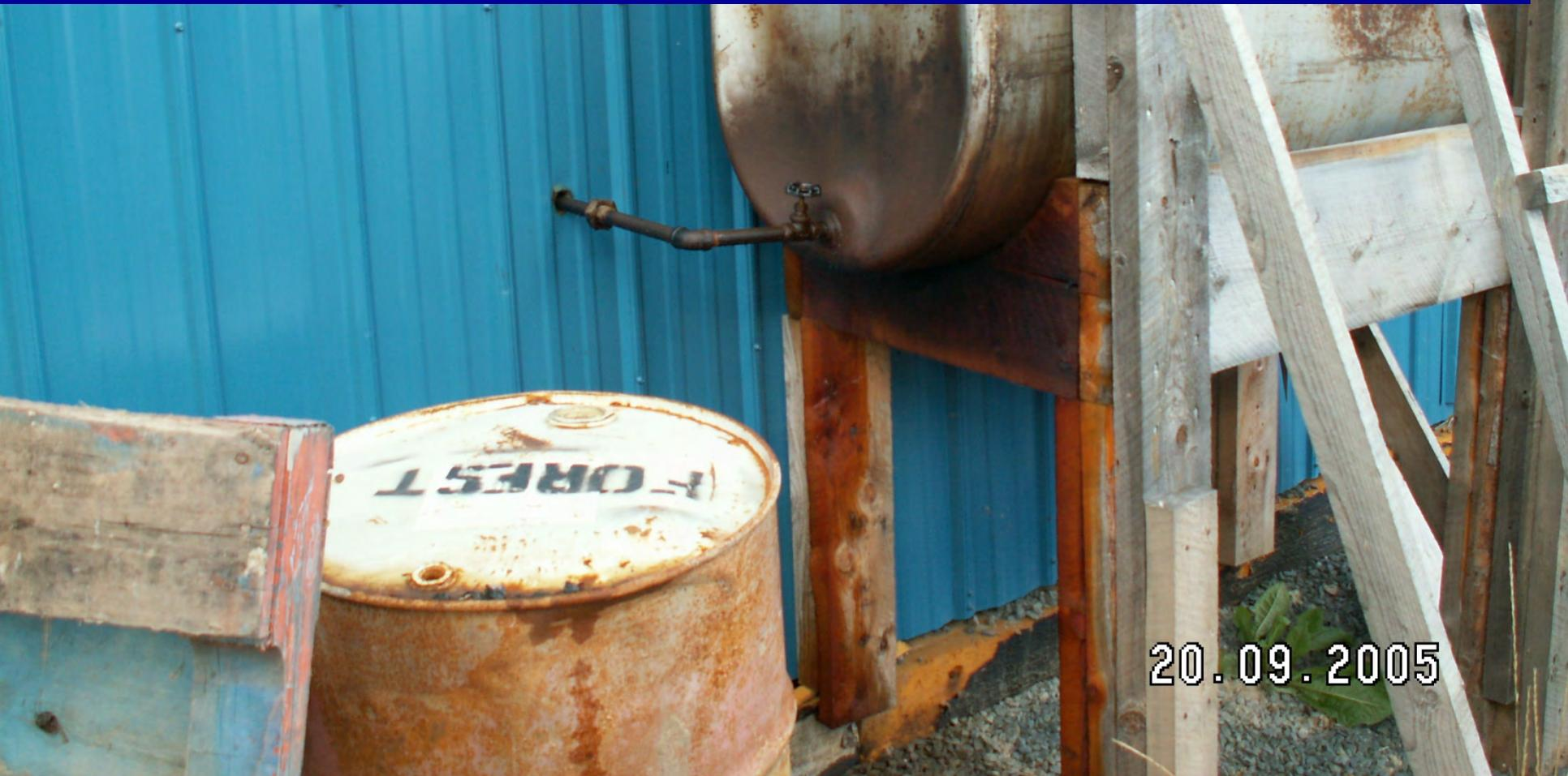
Tank is starting to leak at bottom of the tank
