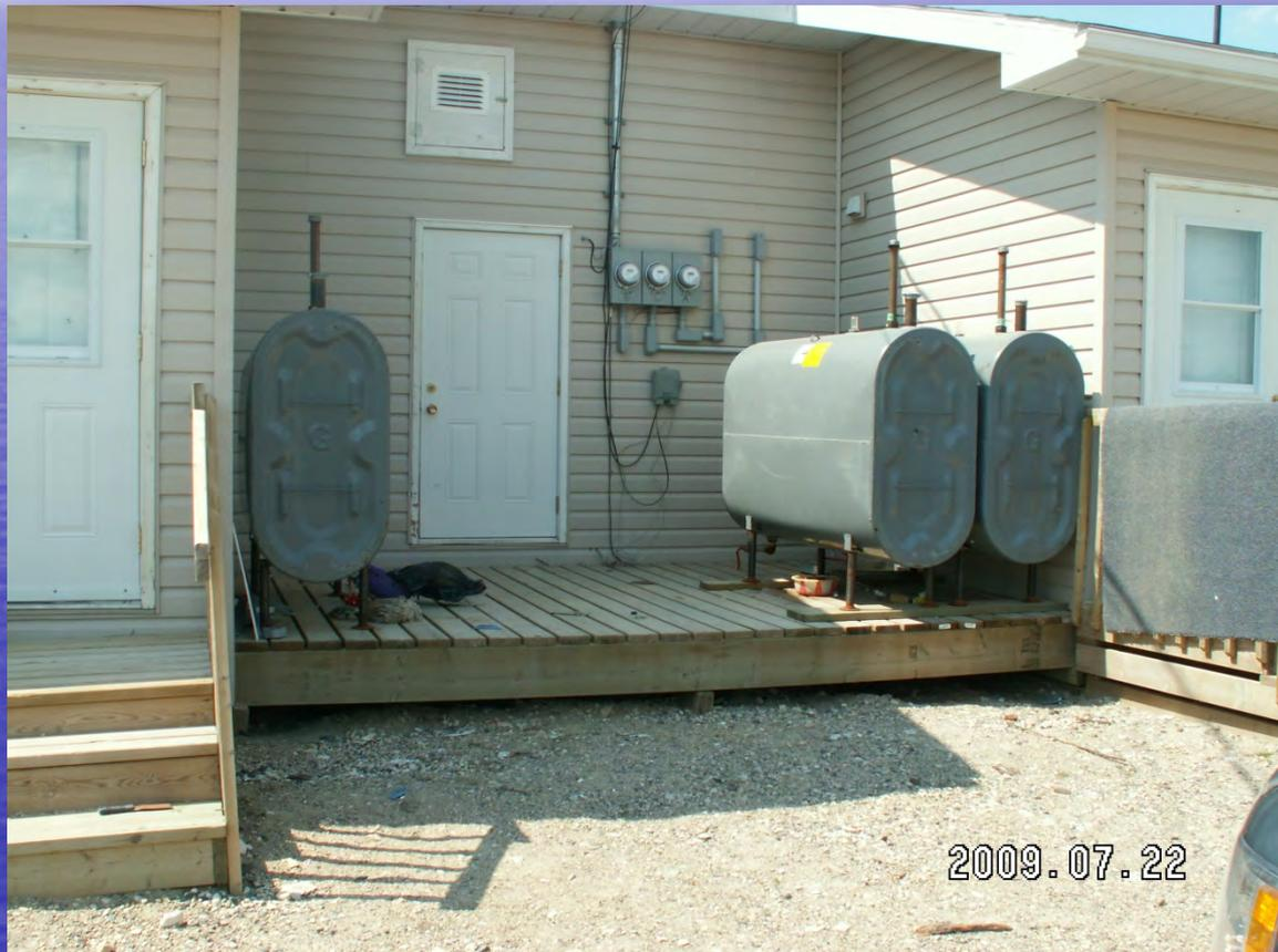
Proper tank installation. Tank is double
