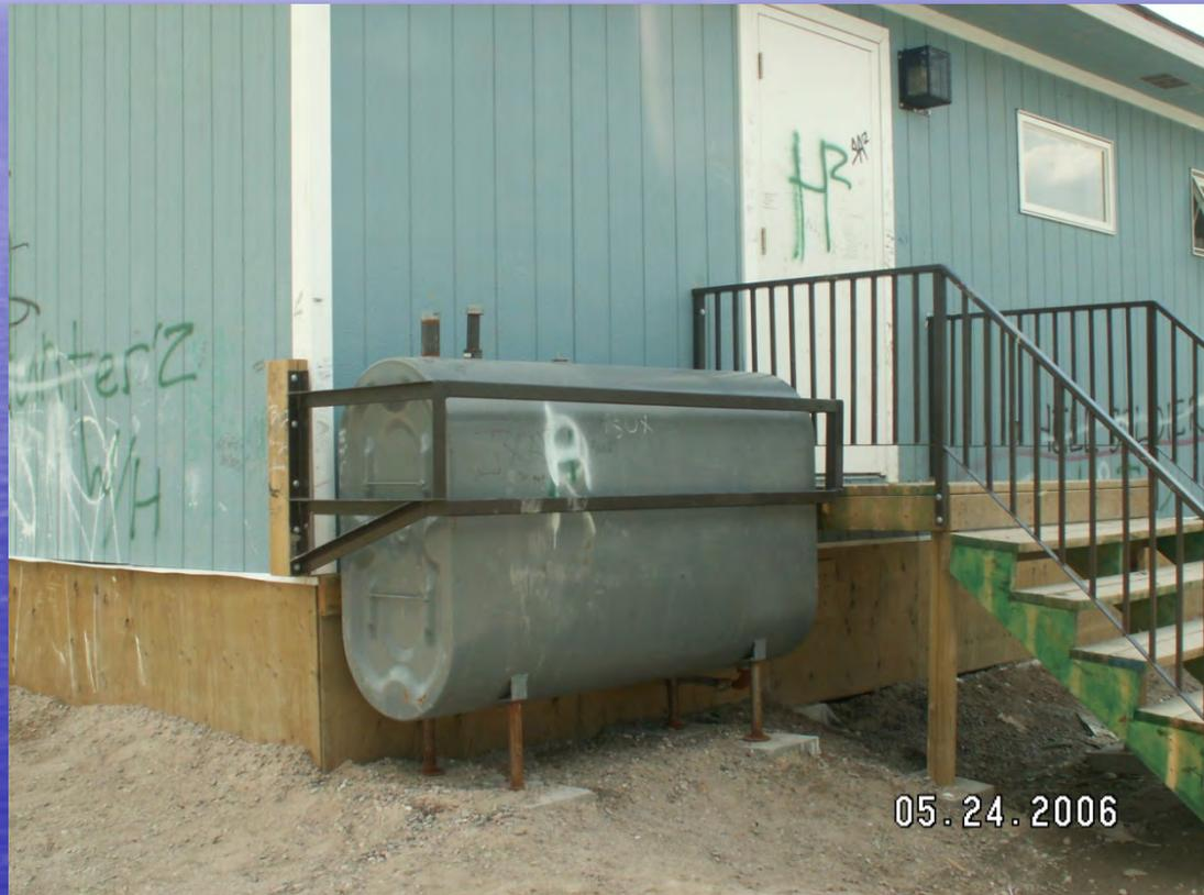
Tank needs to be on a concrete stand. Tank needs to be moved closer to the house.
