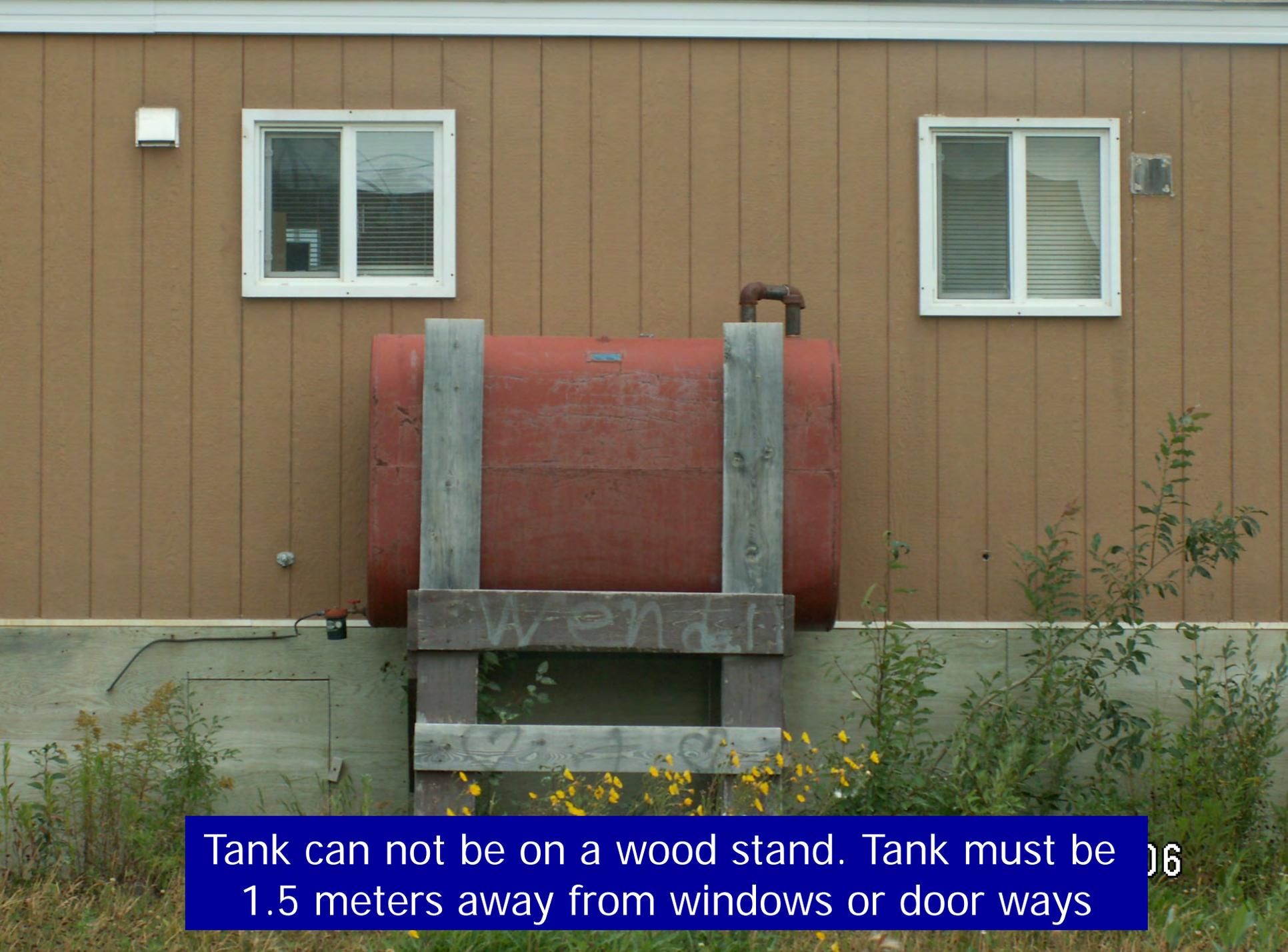
Tank can not be on a wood stand. Tank must be 1.5 meters away from windows or door ways 06
