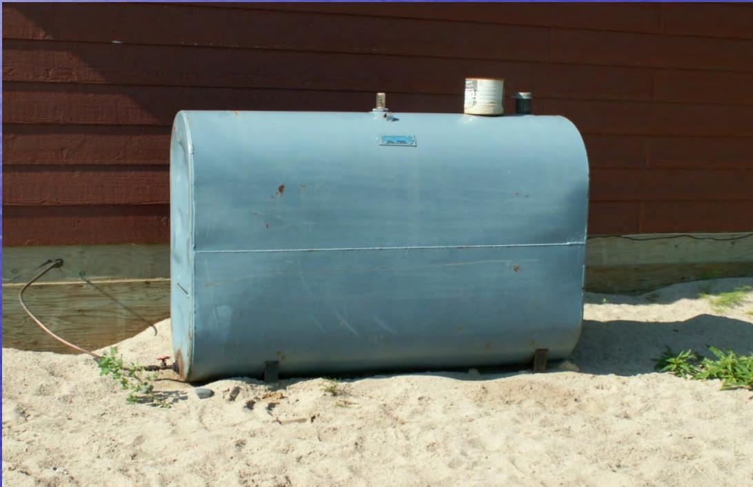
Tank can not be on a wood stand, tank can not be any higher than 12 inches off the ground. Pallets must be removed, they are a fire hazard. Roof must be able to withstand snow load.
