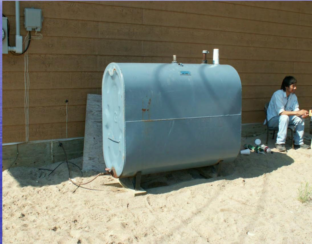
Tank is Settling Into Sand - Tank was not put on a concrete slab as it should be per code
